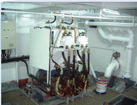
Power pack for steering gear.
